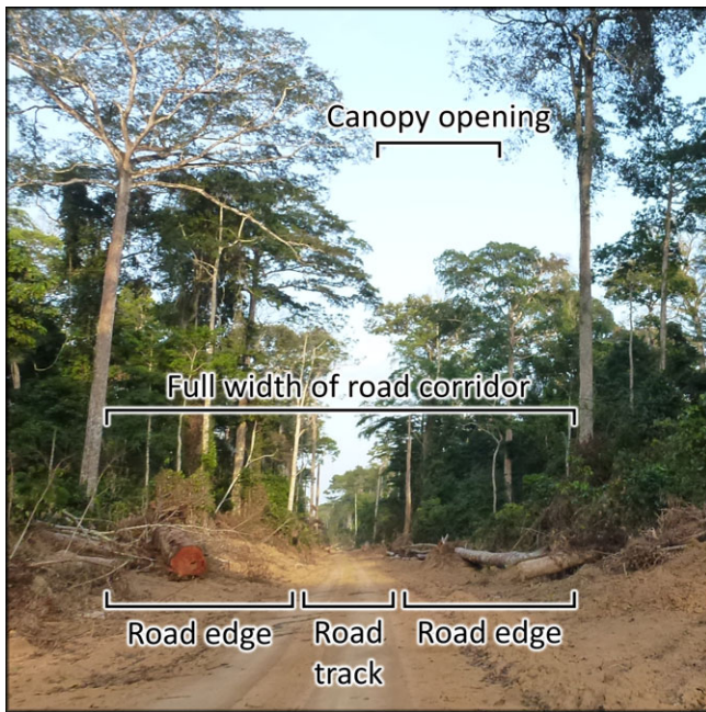
FIGURE 1. Example of a secondary logging road in Republic of Congo annotated with cross-section measures and their respective names used in the text.
